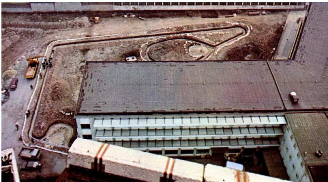
Fig. 3 – Cable trench during laying 1
